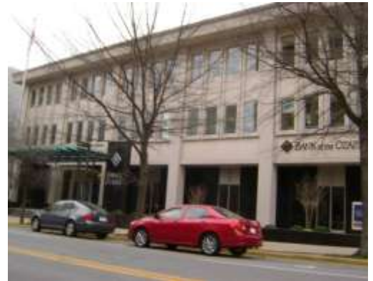
Compliance Networks Data Center in the decommissioned Federal Reserve Bank Building in Little Rock, Arkansas
